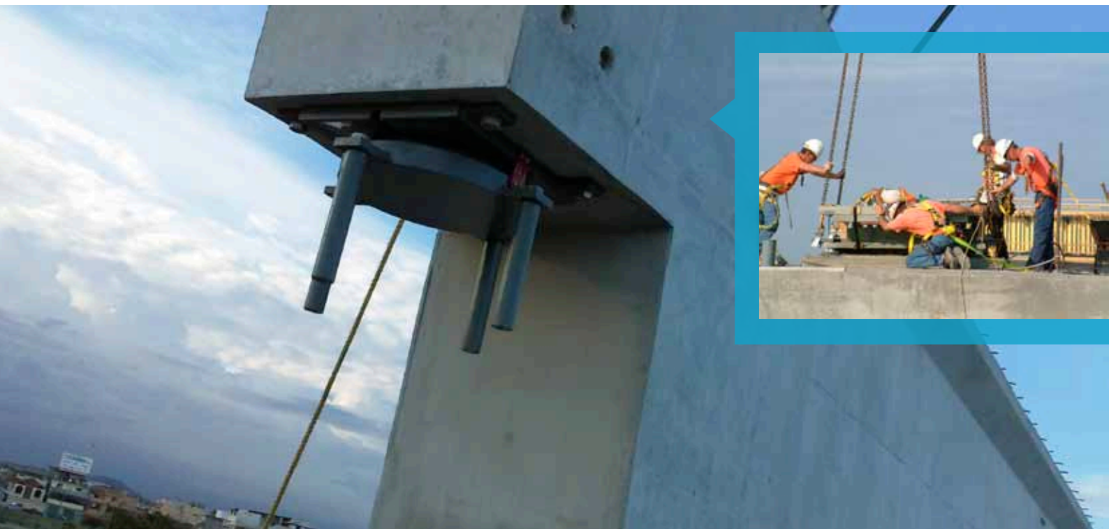
Figure 1 – Detail of Bearing anchorages and installation components
